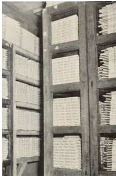
(11) Seasoning: Seasoning gives dimensional stability of the stock. It is one of the key processes and can not be neglected.
