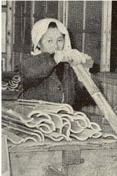
(1) Selection: Pieces of bamboo, which is the main material for slide rules, undergo quality inspection.
