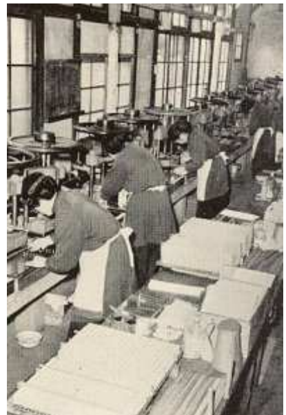
(6) Sheet of Celluloid is glued and pressed. Student rules are not covered with Celluloid on all sides, but are treated with a hard vanish.
