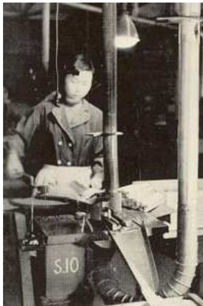
(5) A block is split in half using circular saw, thus making two slide bars at the same time.
