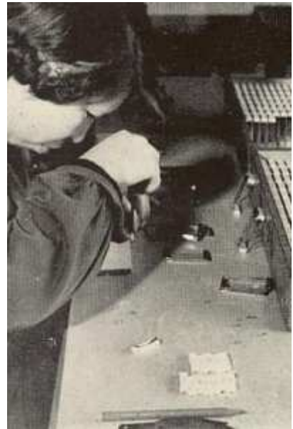
(15) Assembly of two-sided cursors: Two sided cursors are the most difficult to assemble.
